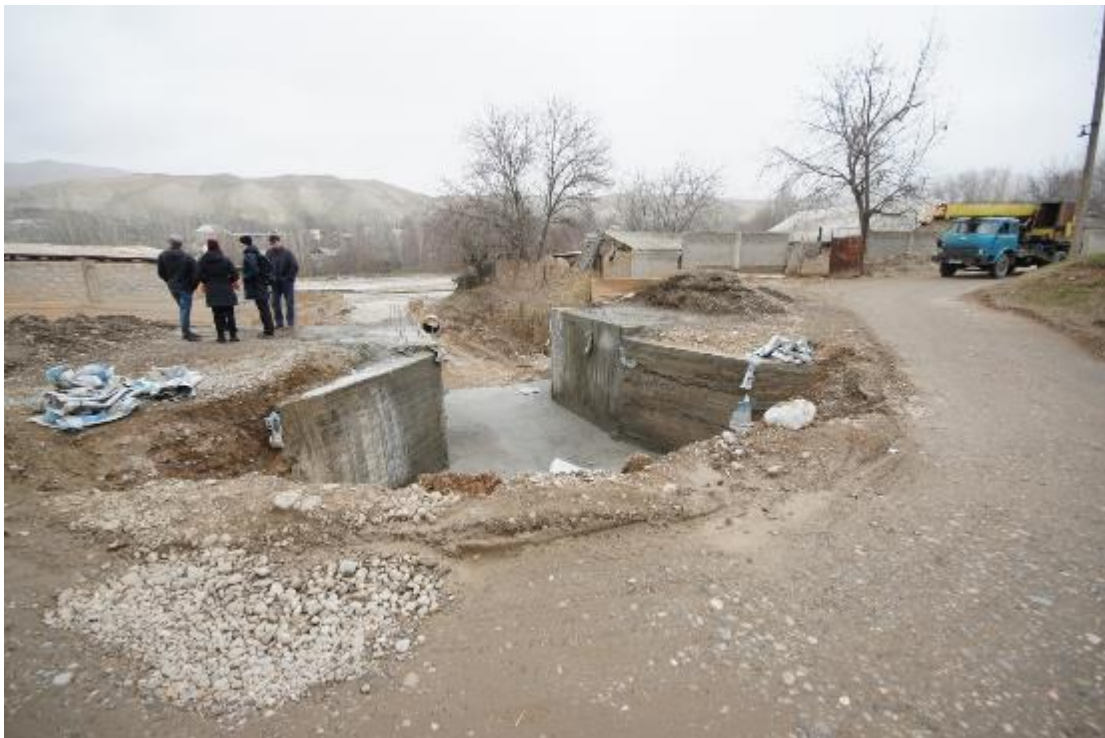
Plate 13: bridge under construction
